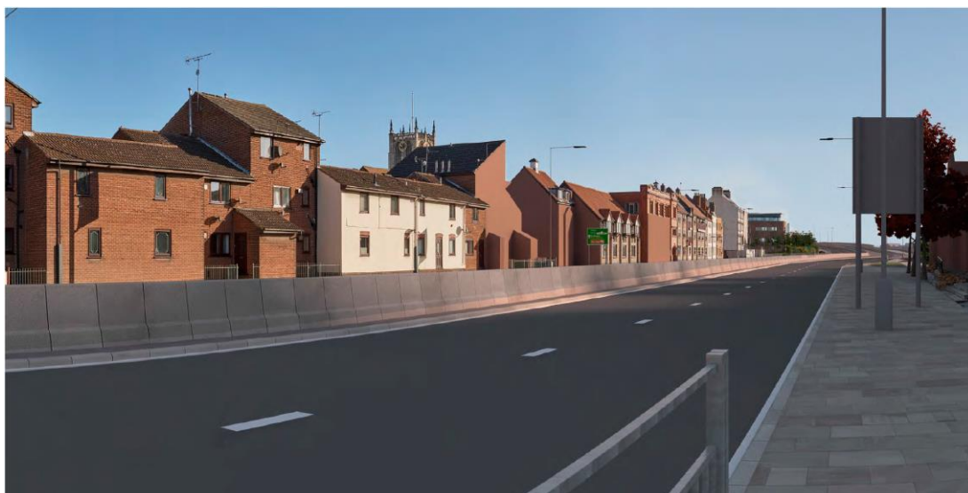
Figure 12: View from the ES showing the central reserve barrier.
